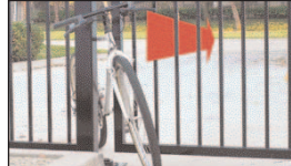
entrapment prevention system reverses gate on contact
